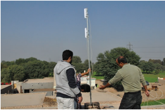
Team installing antenna for connecting the village.
